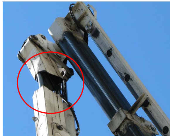
Figure 1 Area of jig failure
